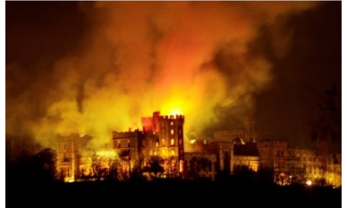
Windsor Castle: 6 mil liters of firefighting water (soil, water system, etc)
